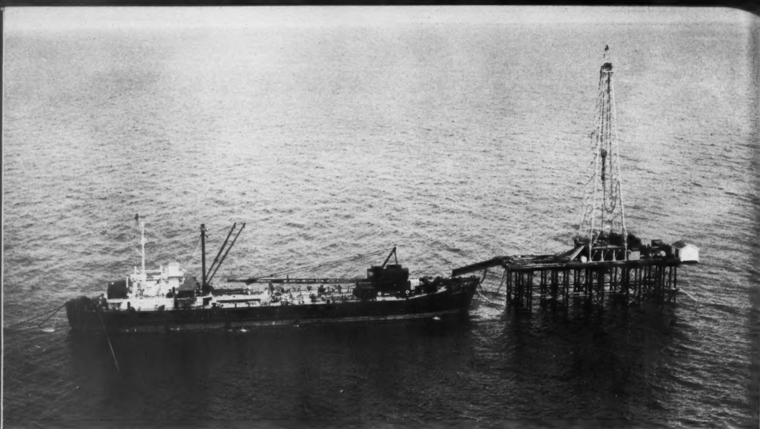
SHIP AND DRILLING PLATFORM form a dramatic, unusual alliance as they join forces in the common cause of supplying heavy demands for oil. Ship serves as floating warehouse, crew quarters; provides well services. Location is at Caminada Pass, off Grande Isle, Louisiana.
